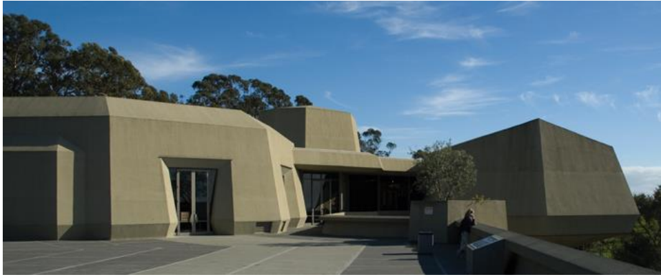
Exterior of the Lawrence Hall of Science Image courtesy of http://www.lawrencehallofscience.org/about/advisory_council
