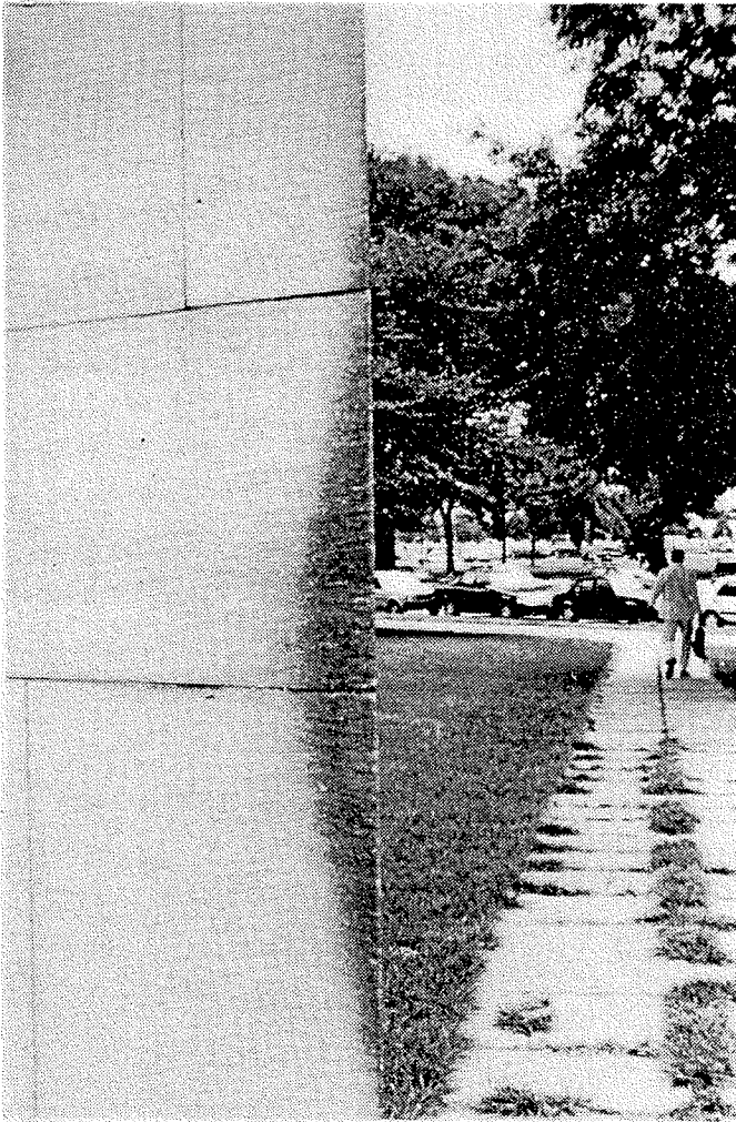
Figure 1 Normal Distribution of Visitors' Hand Prints on East Wing of National Gallery, Washington D.C. (Photo courtesy of Stephen Bitgood)
