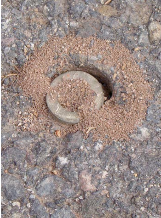
Figure J-5. Ants tunneling around and perhaps undermining sides of markers.
