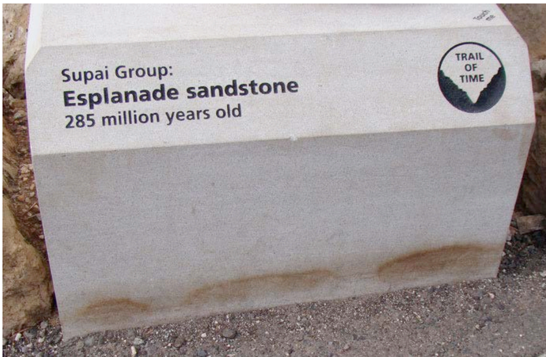
Figure J-15. Some plinths are stained by decaying plant remains, and some are chipped (near center of lower edge of sloped face).
