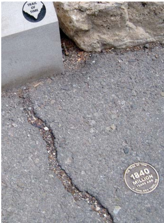
Figure J-3. Trail asphalt cracked in places.
