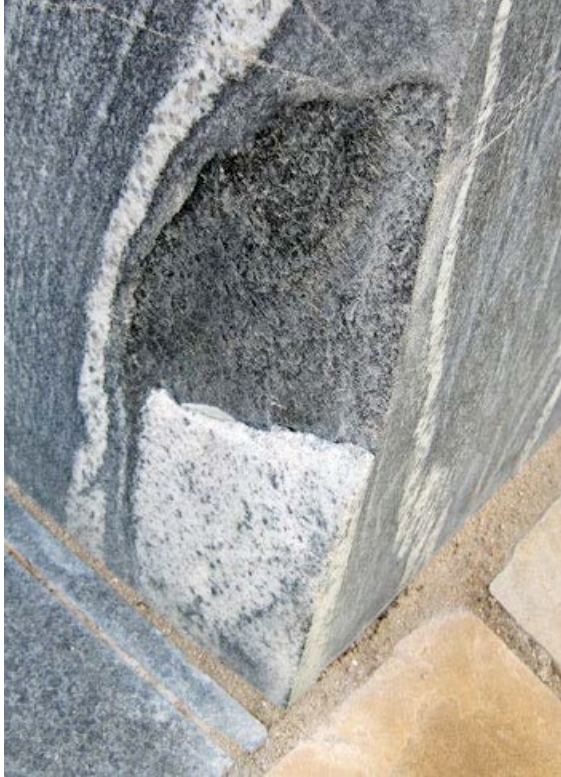
Figure J-9. Broken rock at back corner of the Time Zero portal.
